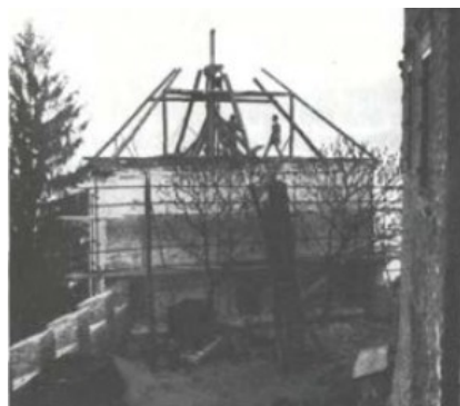
Betonski venec rondele in novo ostrešje
