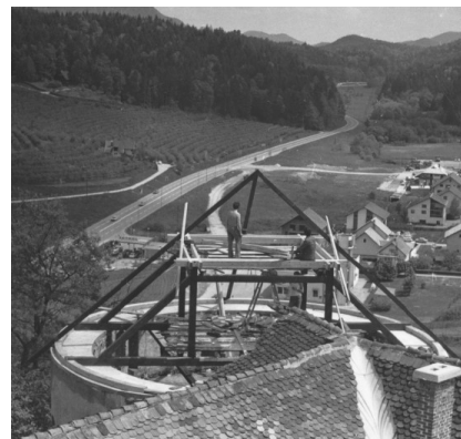
Betonski venec rondele in novo ostrešje
